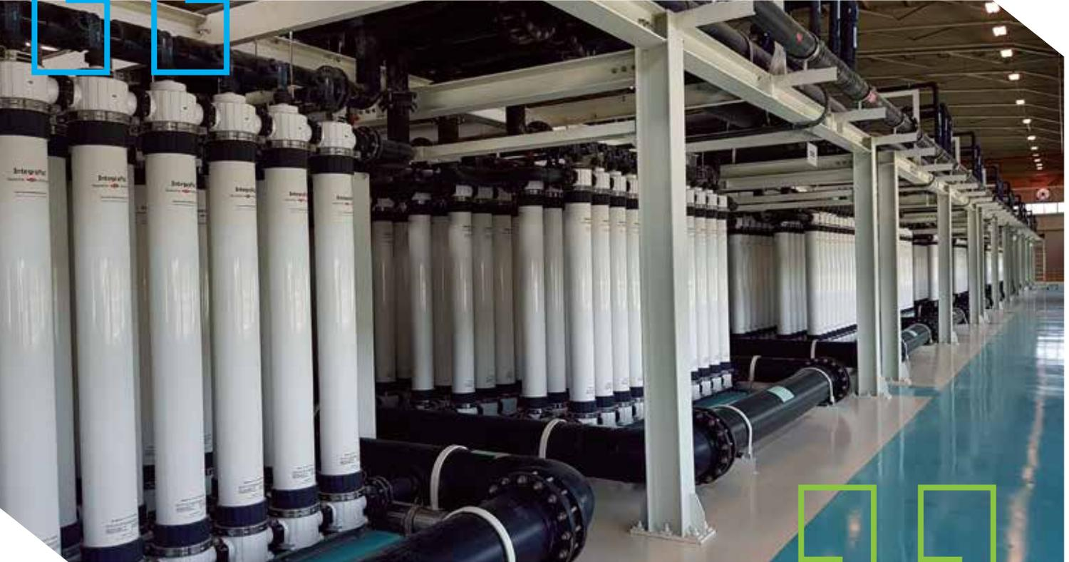
Ultrafiltration (UF) modules has a pore size of 0,02 micron, therefore particles larger than this pore size is removed by the UF membrane, including viruses and bacteria. Ultrafiltration Systems are perfect treatment method for SS (Suspended solids), TOC (Total organic carbon), turbidity, bacteria, viruses and other microorganisms without causing any change in chemical characteristic of the water.
