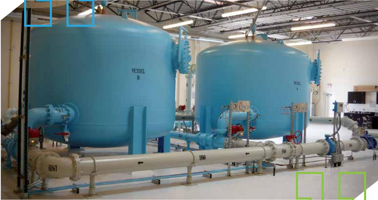
These filters are normally used to remove suspended solid substances that cause turbidity in water. Their operation is very simple and allowing water to pass through several layers of quartz (sand) and, possibly, a layer of anthracite. The water passes through the filtering part, moving in the top-down direction, and during the process the substances retained on the first upper layer of sand increase filtration efficiency in the subsequent layers.
