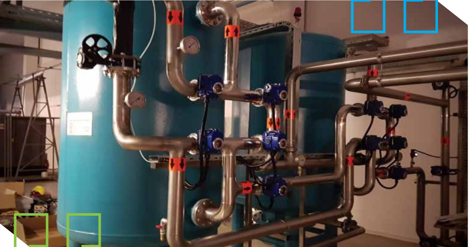
How iron and manganese are removed depends on the type and concentration of water, and this helps determine the best procedure and treatment system. Iron and manganese can be present in water in one of three basic forms: dissolved, particulate and colloidal. The predominance of one form over another is depend on water's pH. The two most common treatment methods are removal by oxidation/filtration and adsorbing onto ion exchange resins.
